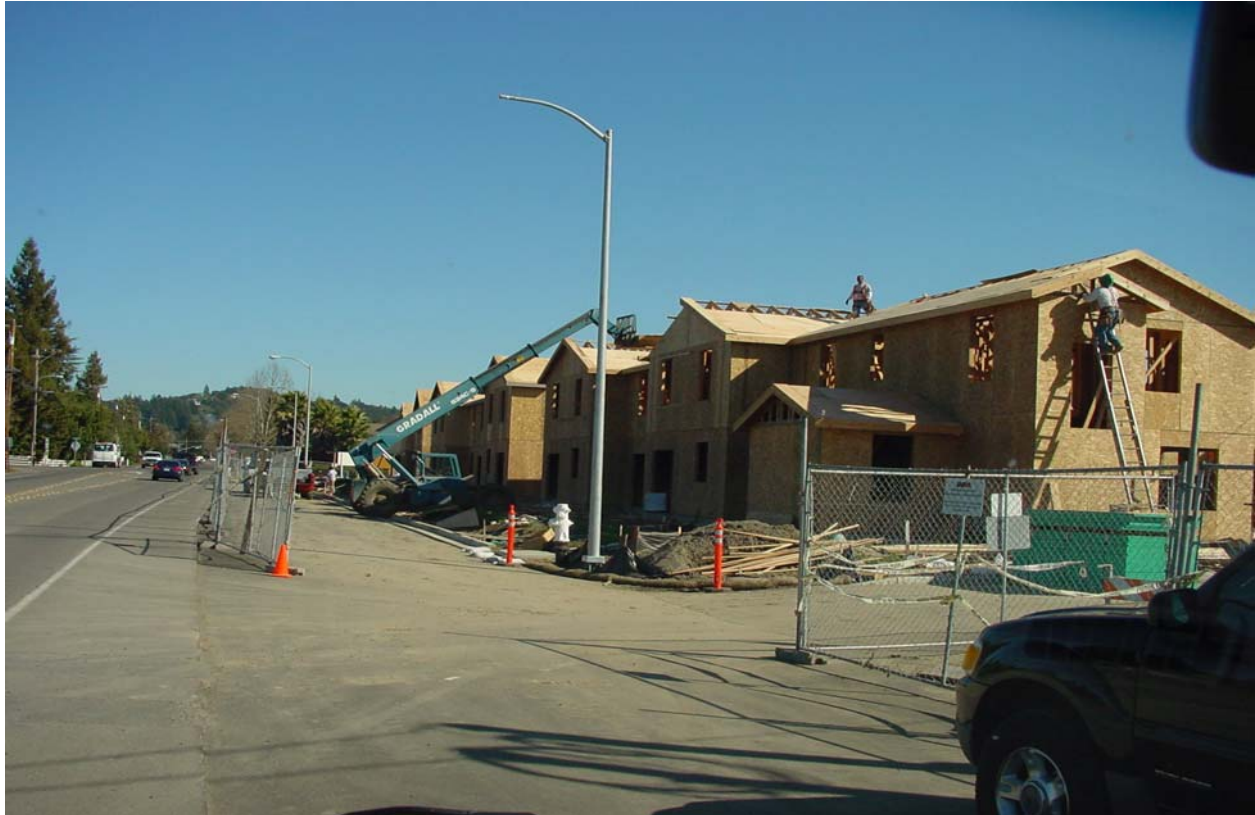
Housing Construction Site Courtesy of Kurt Bauer
