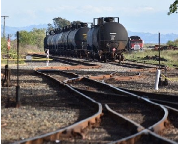
Figure 5: Tank Cars in Schellville
